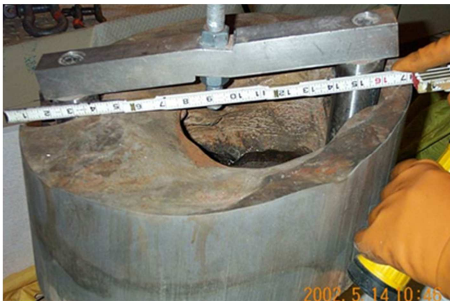
Figure 5.4: Davis-Besse Reactor Pressure Vessel Head deterioration.
