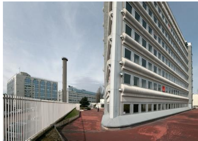
ENSTTI Headquarters Fontenay-aux-Roses, France
